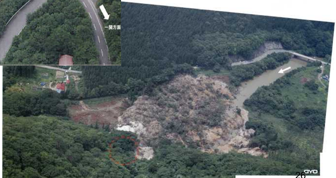
A River Dammed up by Slope Failure Dammed A River
